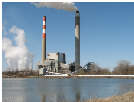
Harding Street power plant Source: IPL
